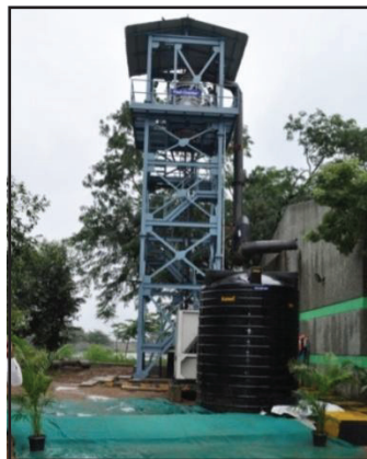
Flash Chamber @11 m height
