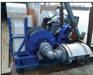
Fabrication of Base frame and installation of New CTD winch
