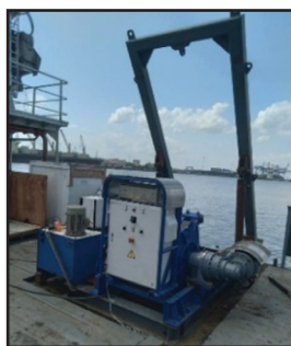
CTD winch A-Frame installation
