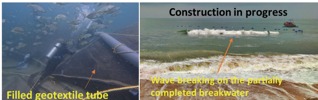
Construction of Submerged breakwater made of geosynthetic tubes
