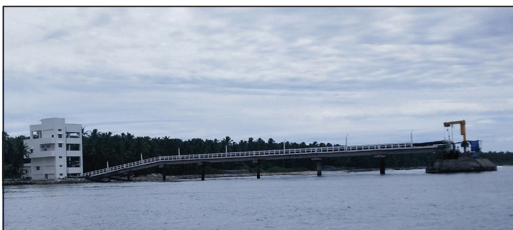
Views of the Sump, Trestle and Plant building of Kalpeni LTTD Plant
