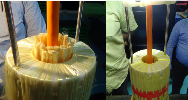
Making the Cable Termination ready
