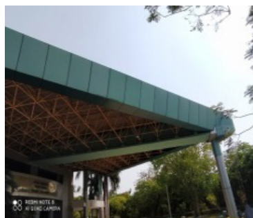
ACP Alco bond composite panel roofing sheet work at entrance of Auditorium
