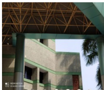
ACP Alco bond composite panel roofing sheet work at entrance of Auditorium
