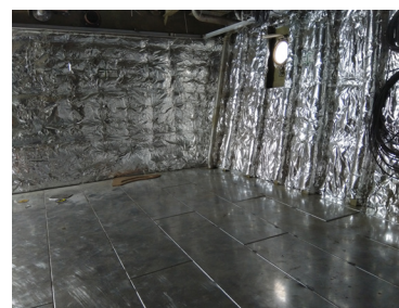
Laying & Fixing of insulation, Wall Panels & Floating Floors in accommodation areas
