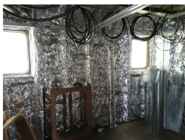
Laying & Fixing of insulation, Wall Panels & Floating Floors in accommodation areas
