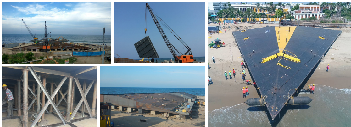
Construction and Launching of the Steel Reef
