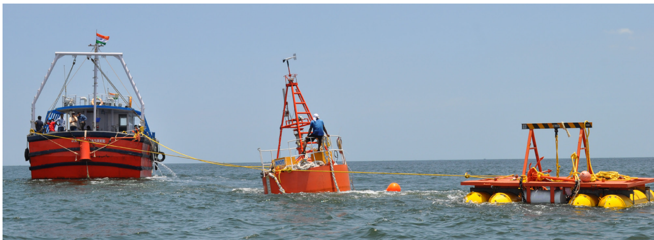
Towing of the buoy to site
