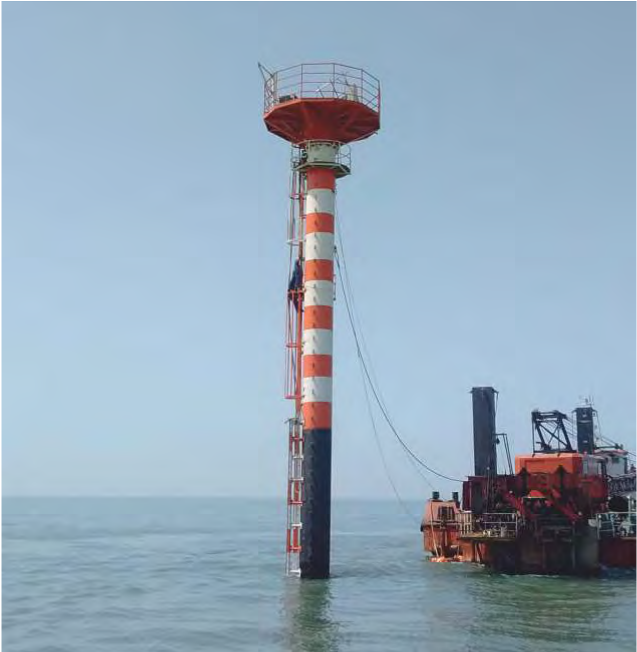
Supporting substructure for LiDAR platform installed at Gulf of Kambhat
