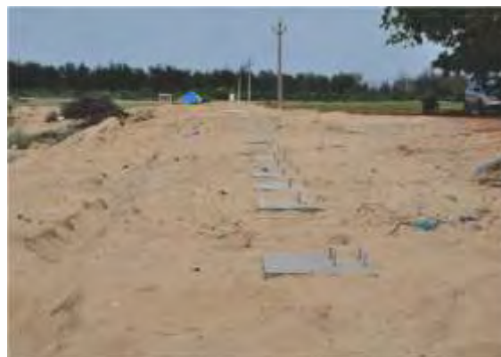
Construction of foundation for chain link fencing at Pamanji
