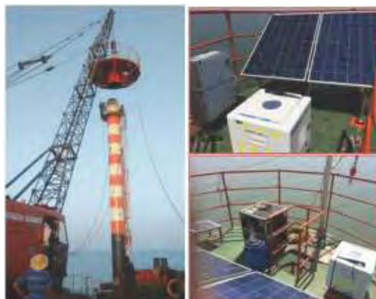
Installation of Substructure for Offshore Wind Measurements
