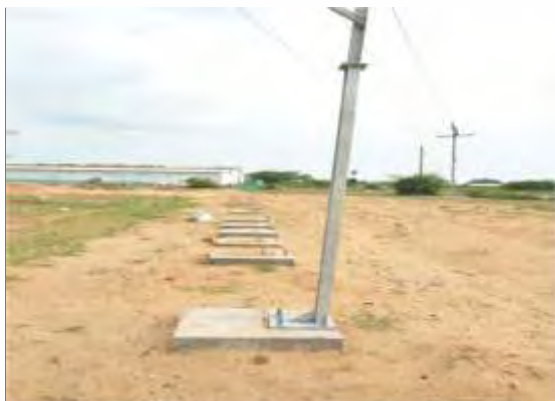
Construction of foundation for chain link fencing at Pamanji
