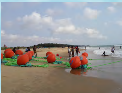
Preparation of cage mooring grid at Tuplipalem
