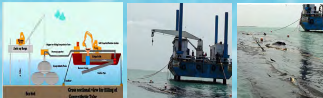
Filling of geo-synthetic tubes at site
