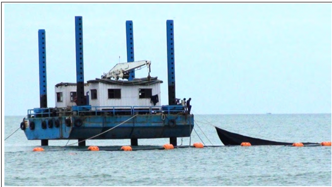
Installation of geosynthetic tube for submerged breakwater at Kadalur Periya Kuppam
