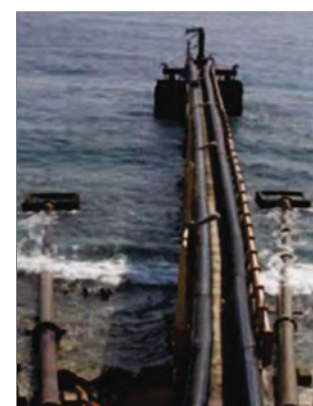
b) Replaced GFRP outfall pipe at Minicoy Island
