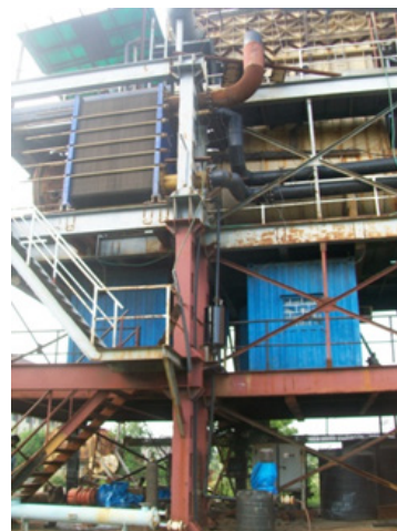
LTTD with PHE as condenser
